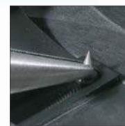
Replacing the discharger electrodes
